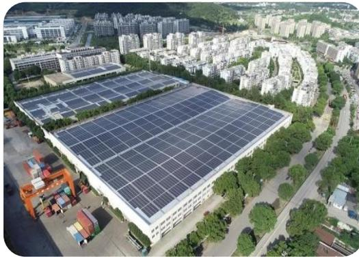
**Construction Plan:** Establish distributed power generation system by laying rooftop photovoltaic in the park for consumption and excess to the grid. **(Under construction)**
